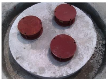
(c) 刚度调节装置安装
